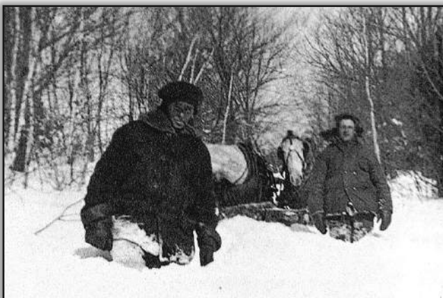
Sometimes the Town used a homemade horse-drawn wood-shod sled with a land plow and mold boards strapped to it. Horses would use it to plow a path so it was easier going. The picture shows two men breaking trail for the horses and plow sled on Town Farm Road near the intersection with South Road.
