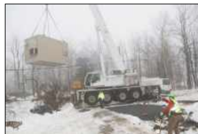
Installation of Heath’s fiber hut in town center. The hut is the central point of connection and distribution for Heath fiber.
